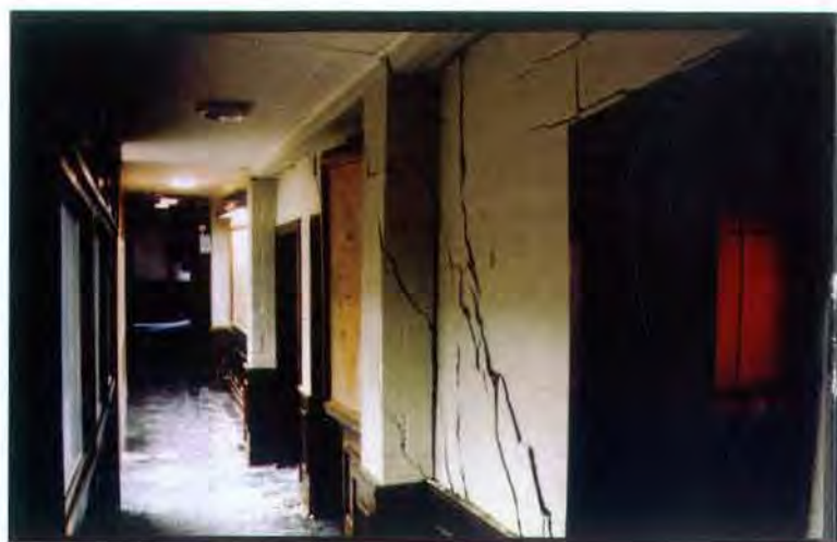
Figure 4. Building damage due to loess collapse.
