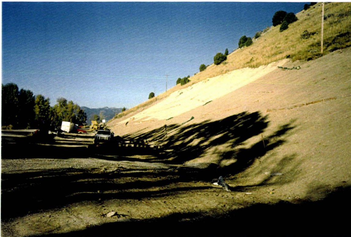
October 8, 1998: Placing erosion control fabric at the School Pit, LEBS in place
