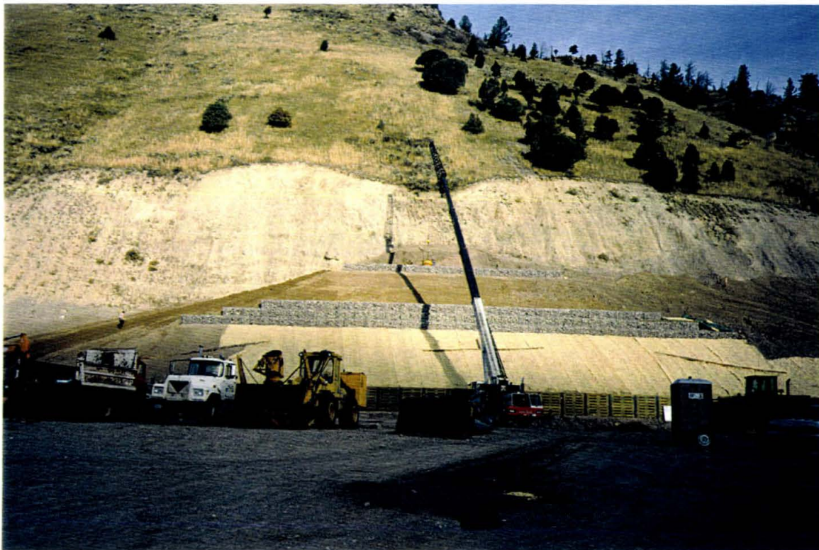
October 14, 1998: Filling gabion baskets on uppermost tier at Simon Pit
