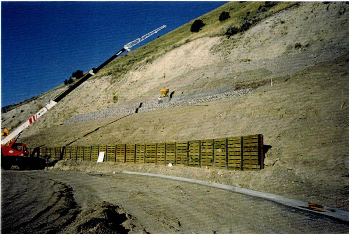
October 8, 1998: Filling gabion baskets at Simon Pit, SPLR curb and gutter in place
