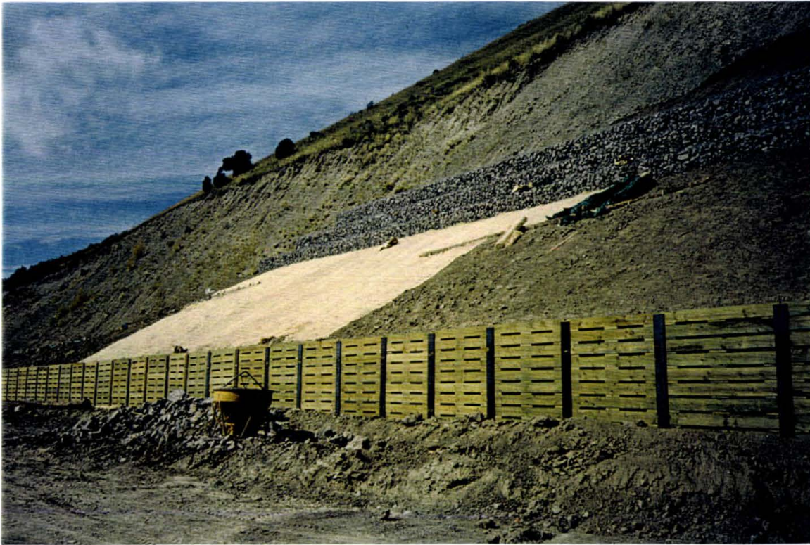
October 10, 1998: Placing erosion control fabric between retaining walls at Simon Pit
