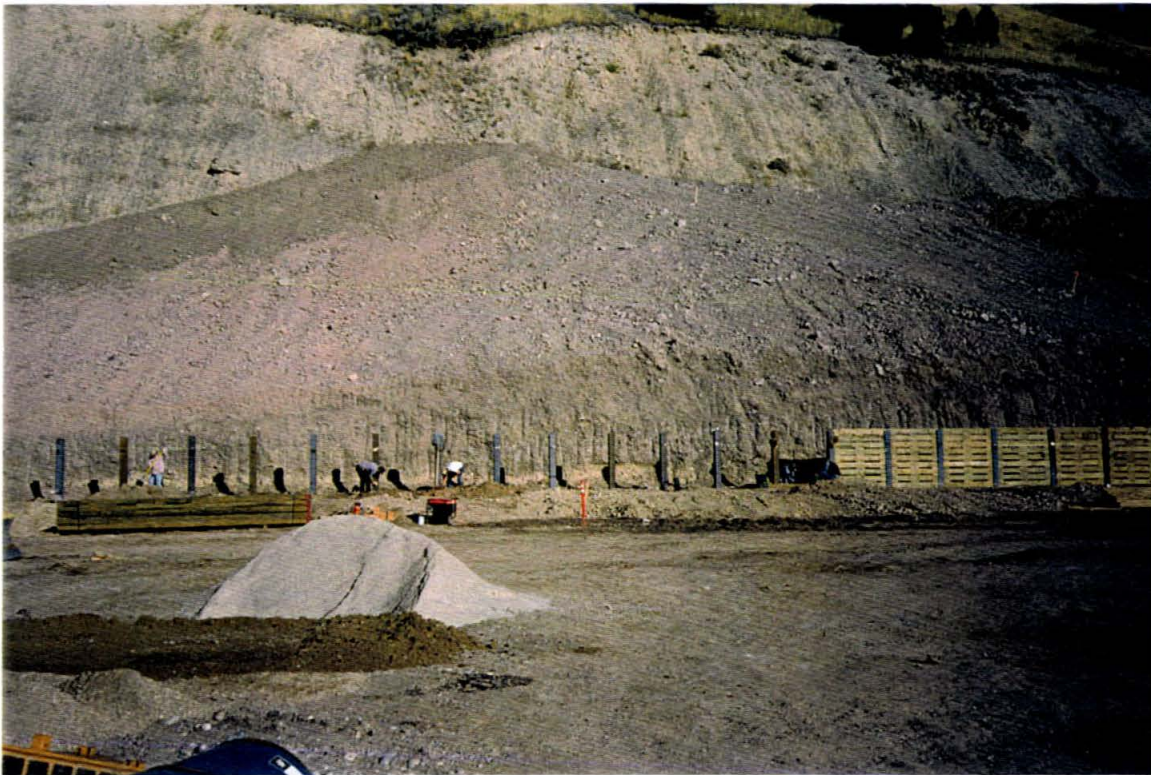
September 24, 1998: H-pile retaining wall at Simon Pit
