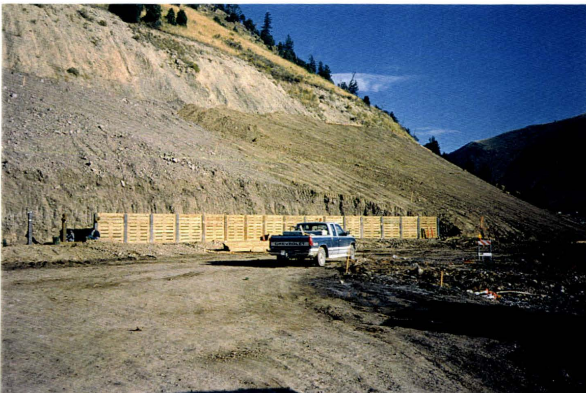
September 17, 1998: H-pile retaining wall & topsoil placement on the northeast corner of the Simon Pit
