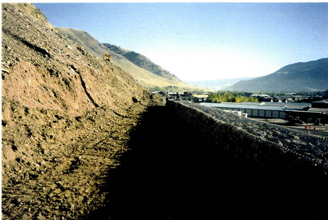
October 8, 1998: Gabion basket retaining walls at Simon Pit
