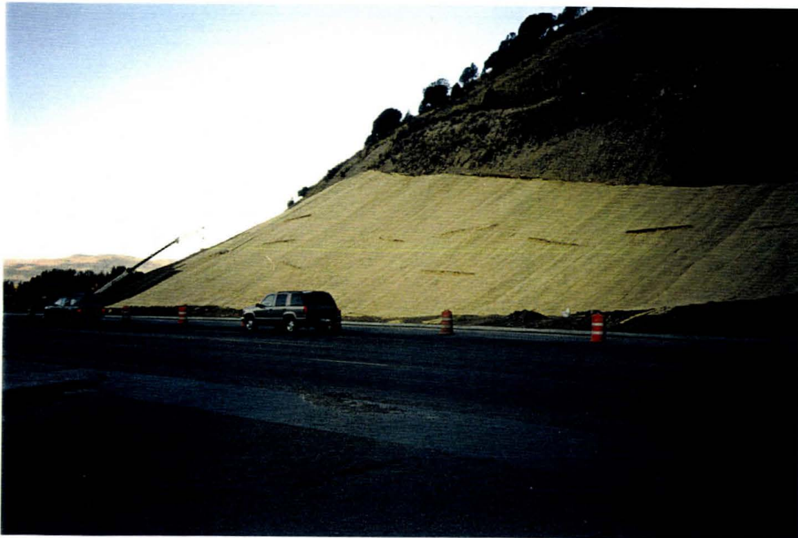
October 9, 1998: Erosion control fabric on northeast corner of Simon Pit
