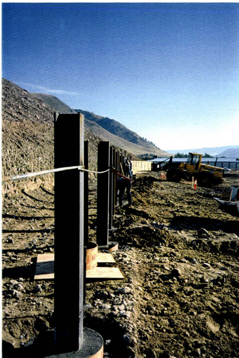
September 24, 1998: Constructing H-pile retaining
