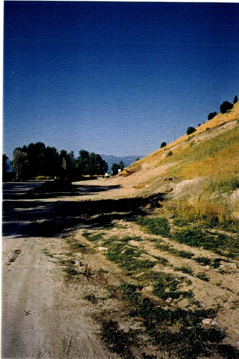
September 12, 1998: West end of School Pit Silt fence in place, Fill being placed
