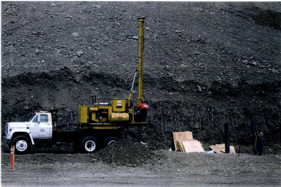
September 18, 1998: Drilling holes for H-pile Retaining walls Simon Pit
