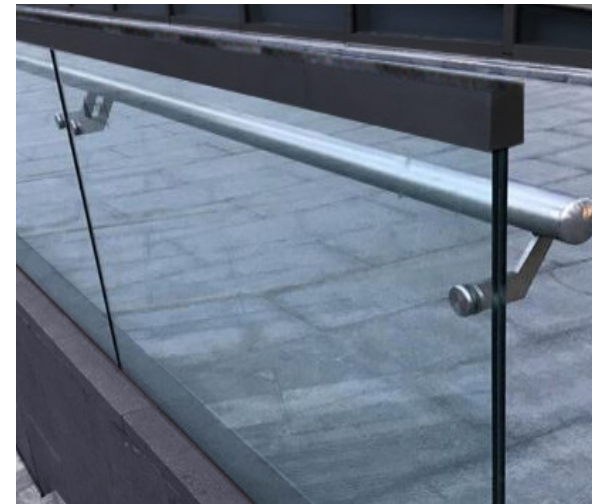
INDUSTRIAL STEEL / GLASS RAILING @ POOL AREAS
