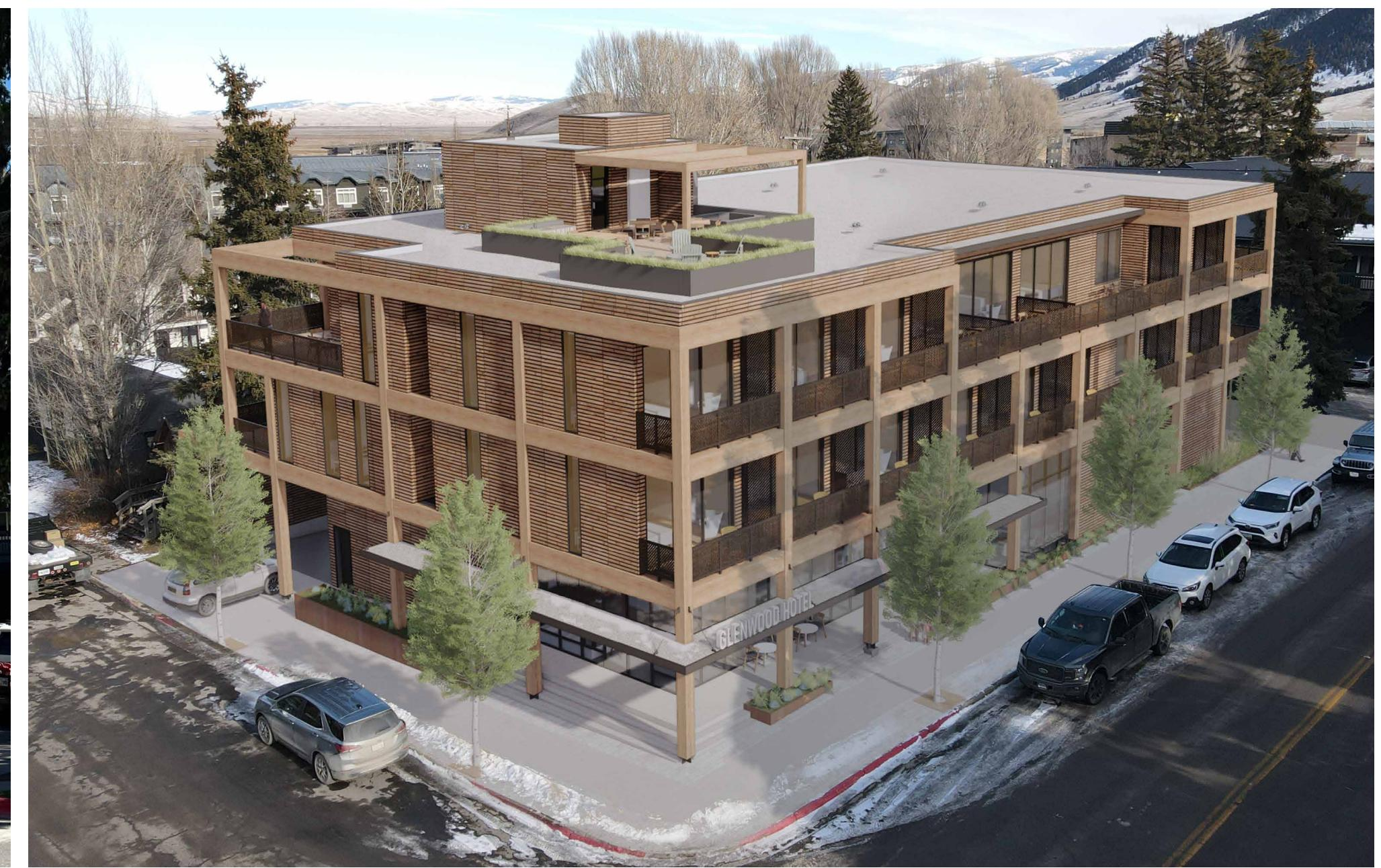
THE DESIGN TEAM BELIEVES THAT THIS OPEN-AIR BEAM EXTENSION ALONG GLENWOOD STREET PROVIDES THE LIGHT, AIR & REDUCTION IN VOLUME THAT THE STEPBACK REQUIREMENTS PROMOTE – WHILE PROVIDING A MORE ELEGANT CORNER SOLUTION THAT TERMINATES THE STRUCTURAL GRID IN A MORE VISUALLY PLEASING MANNER.
