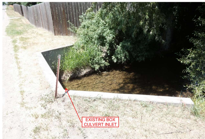
Figure 3. Box culvert inlet
