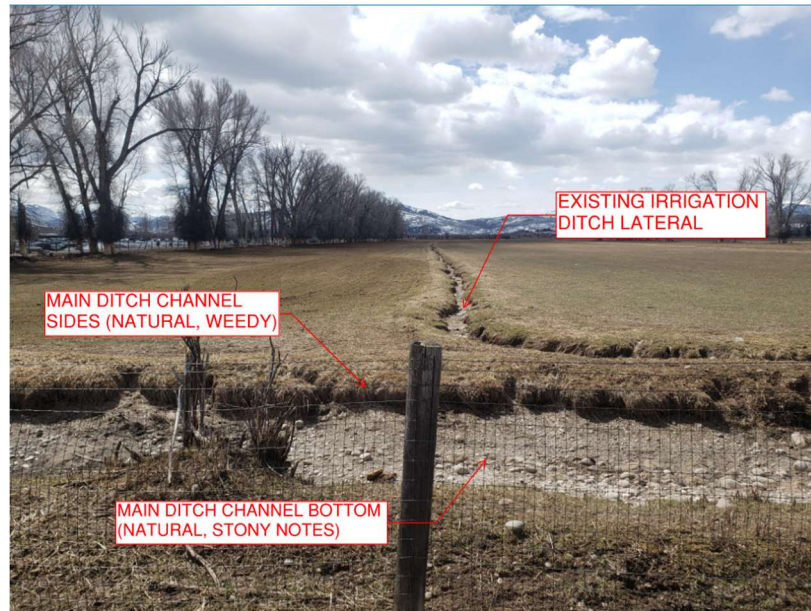
Figure 2. Existing main & lateral channel conditions
