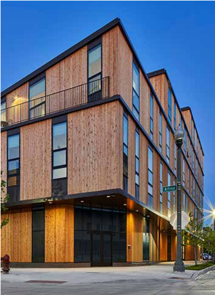
2 CEDAR SIDING EXTERIOR WALLS, LEVELS 2 & 3, & ROOF FASCIAS
