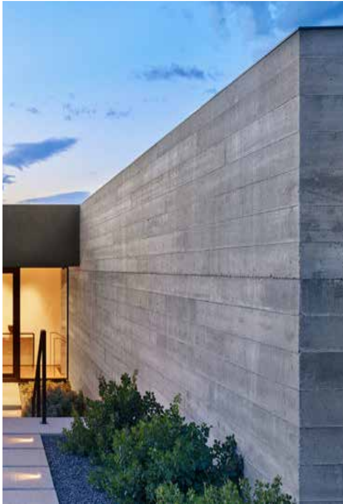
1 BOARD FORMED CONCRETE EXTERIOR WALLS, LEVEL 1
