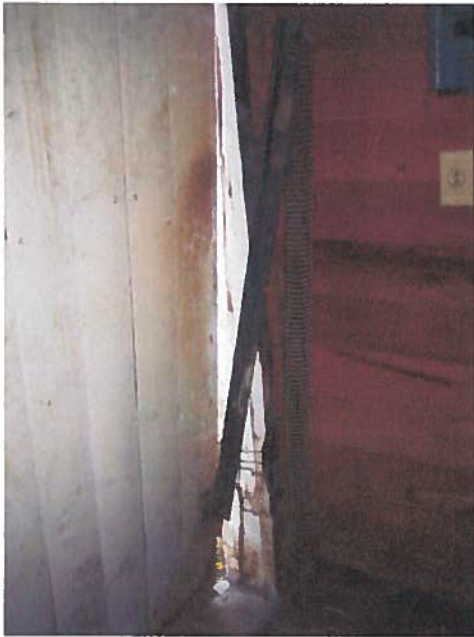
FIGURE 32: The hardware used to raise the 2 overhead doors is old and unsafe.
