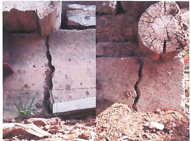
FIGURE 25: These foundation cracks are located on the west side of the building, near the corners.
