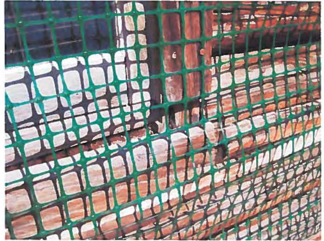
FIGURE 41: The window trim is loose and has started to fall off. Also please note the green mesh over the window.
