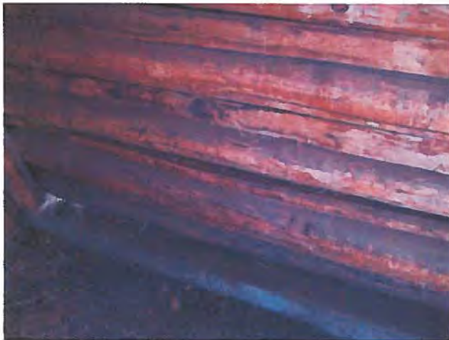
FIGURE 42: The scribed wood chinking on the interior of the building has pulled away from the logs and filled in with dirt.
