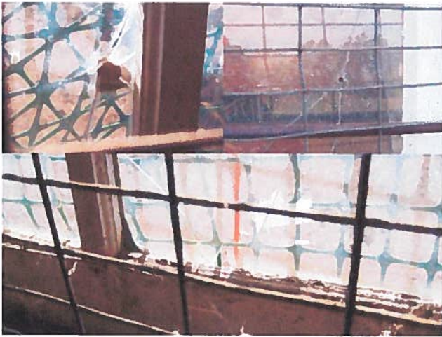
FIGURE 36: A few planes of glass are broken on the ground level.
