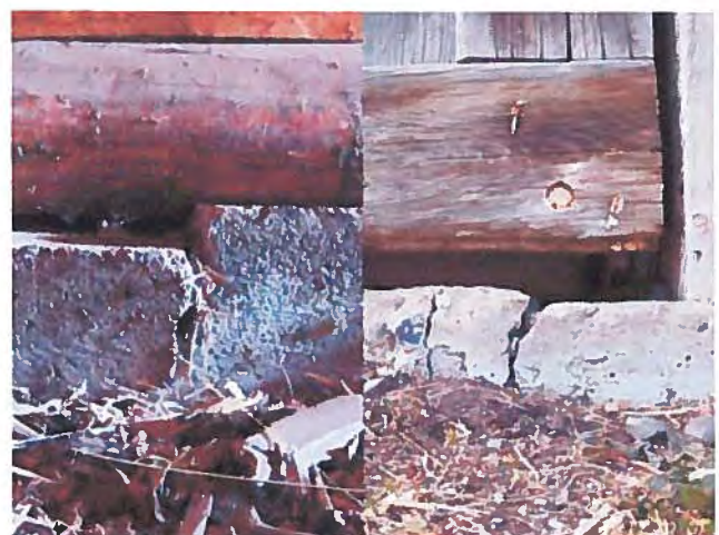
FIGURE 27: The foundation crack on the left is located on the south side of the building. The crack on the right is located on the east side of the building. On the south and east sides of the buildings, grade is covering up most of the foundation, so there may be more cracks that are not visible.
