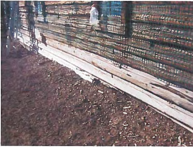
FIGURE 28: The sill log on the south side of the building has deteriorated so much that it is almost completely gone in sections.
