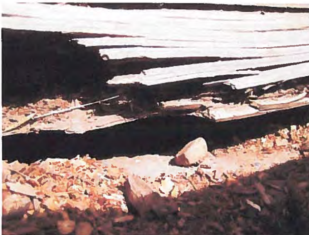
FIGURE 30: A close-up look at the sill log on the south side of the building from the exterior.
