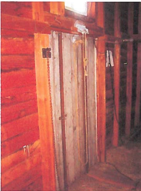
FIGURE 38: The hayloft door is in good condition, however the hardware used to lower it needs replacing.
