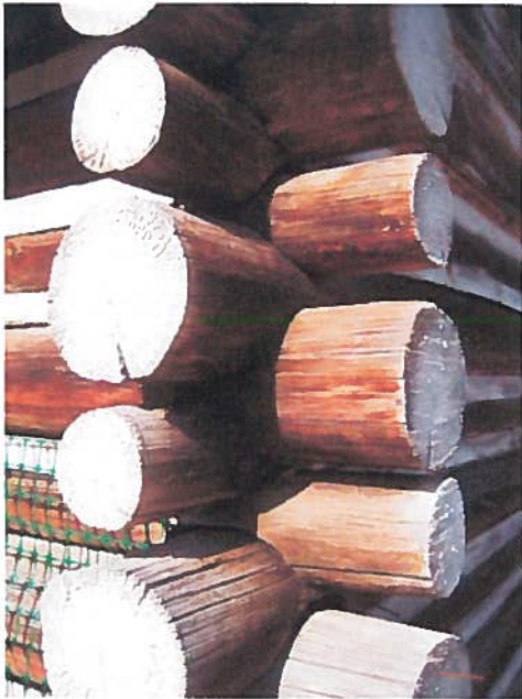
FIGURE 8: Corner detail of the horizontally-laid, corner saddle notched log construction.
