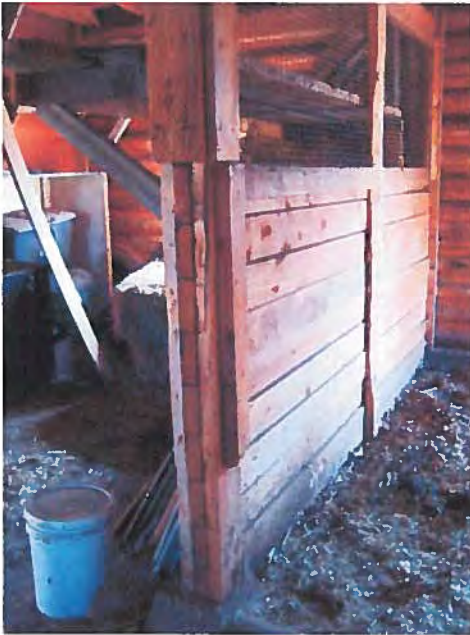
FIGURE 40: The 2x6's that create the stall wall are built-in to the wood post that support the log beams above.
