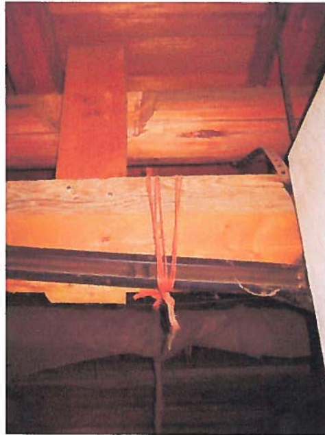
FIGURE 33: Part of the track on the west overhead door is being held up by twine.
