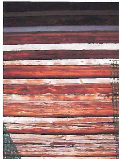
FIGURE 23: This photo is taken on the south side of the building. Higher up, where the roof overhangs blocks the sun, the chinking is still white. Lower on the wall where it gets sun exposure, the paint has chipped off.
