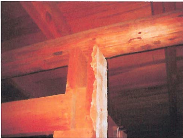
FIGURE 10: One of the wood posts supporting one of the log beams.
