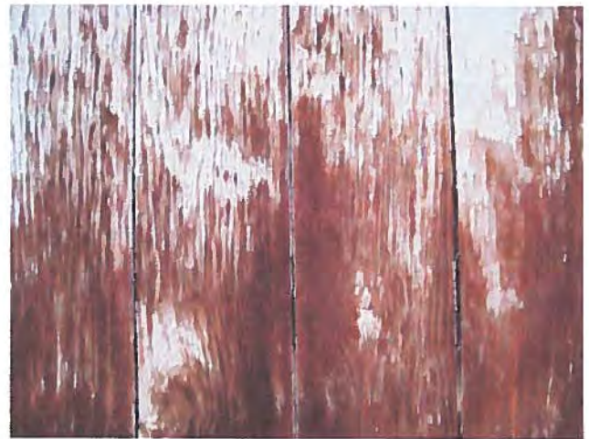
FIGURE 21: Old white paint is chipping off the entry door.
