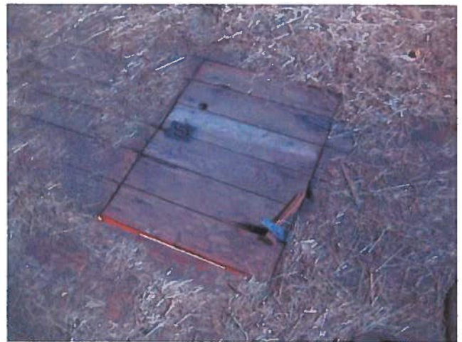
FIGURE 37: The hayloft access hatch, leading from the center aisle, has a broken hinge making it difficult to use.
