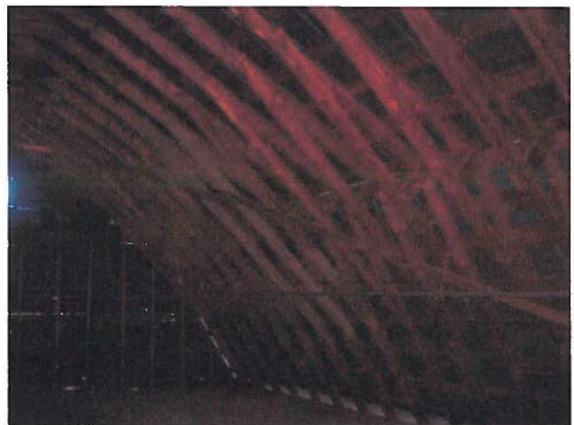
FIGURE 11: Gambrel roof framed with 2x6's.
