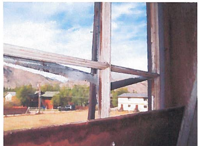
FIGURE 39: The windows in the hayloft are missing glass which was replaced by screen. Also the muntin bars and trim are falling apart.
