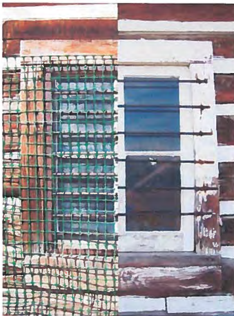
FIGURE 22: The left side of this photo is a window on the south side of the barn, with most of the paint chipped off. The right side is a window on the north side, which still has white paint on it. Also please note the green mesh on the south side.
