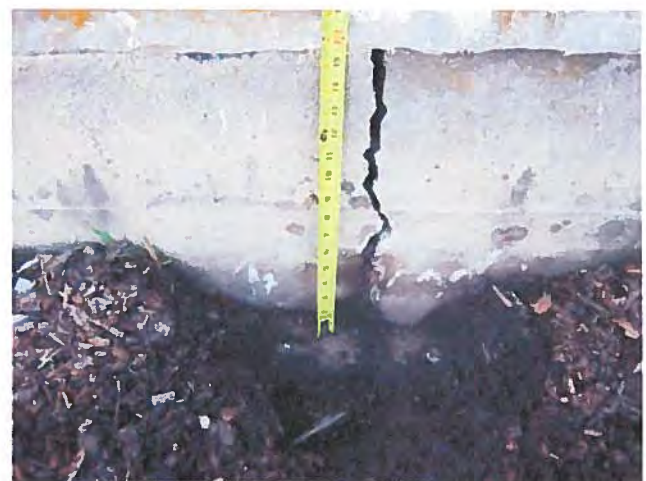
FIGURE 47: A test pit that is dug on the South side of the barn.
