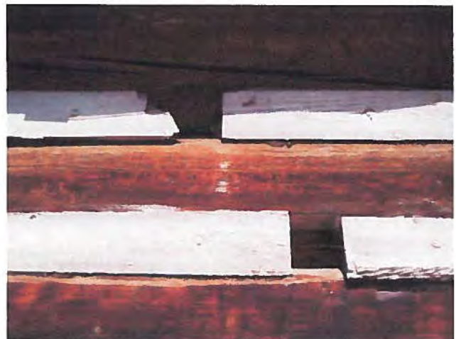
FIGURE 43: The scribed wood chinking on the exterior has broken off in a number of different places.
