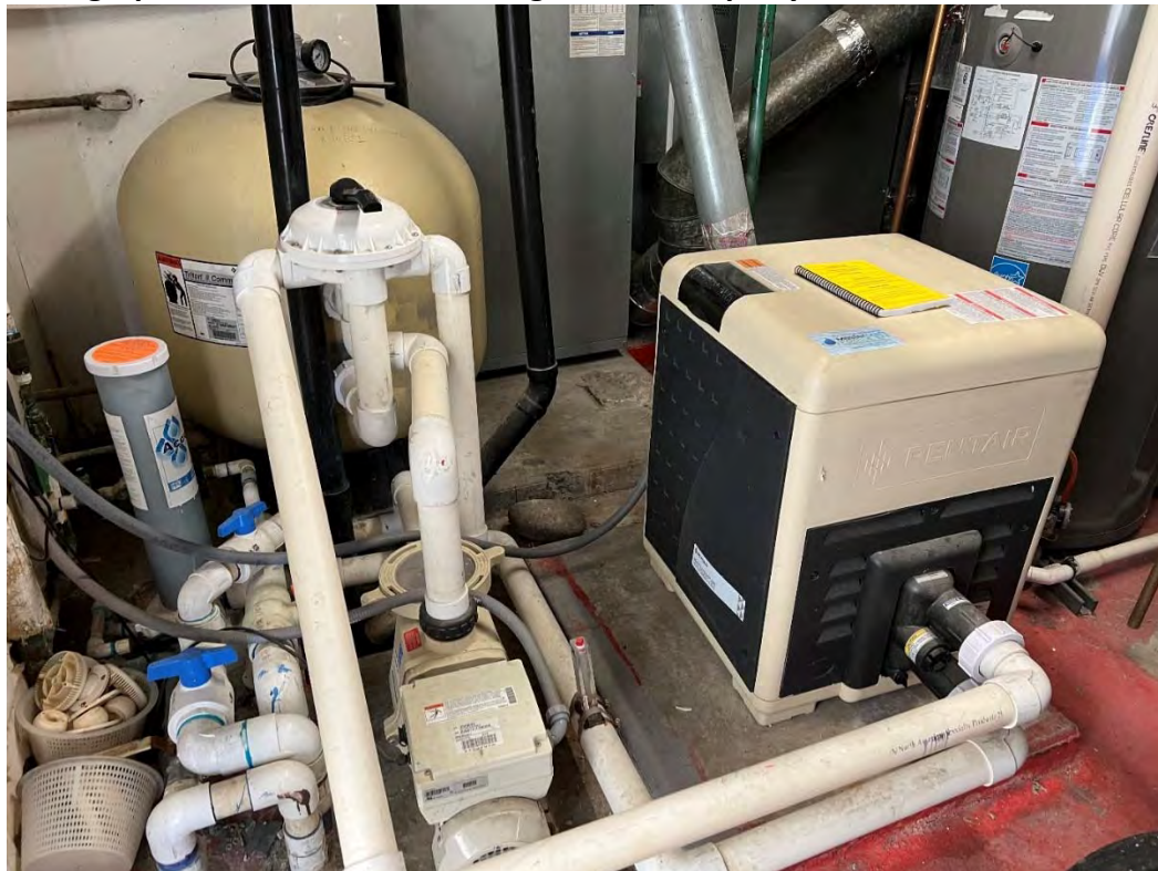
Photograph 14. Pool water maintenance system in the mechanical room.
