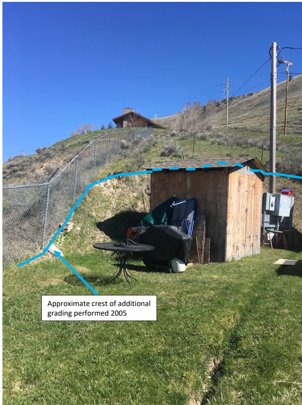
Photo 1 – Photo taken facing NNW near the NW corner of the subject property. Grading that appears to have been performed between 2003 and 2005 is indicated. Photo dated May 2017, C Lane.
