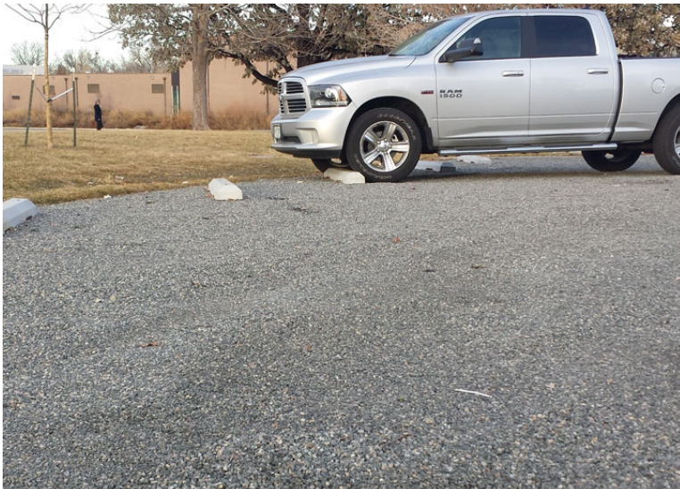
Figure 2 - Gravel Parking with Angled Wheel Stops
