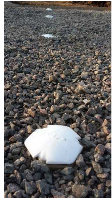
Figure 1 - Parking Space Markers in Gravel
