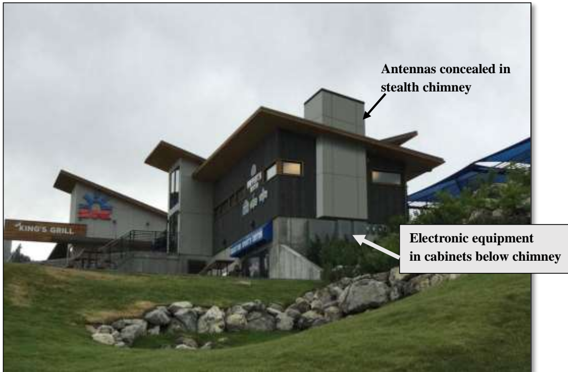
Figure 5: Proposed Stealth Chimney (West Elevation Photosimulation)
