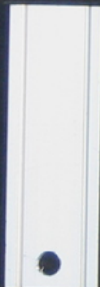
WINDOW CLADDING (CLEAR ANODIZED ALUMINUM)
