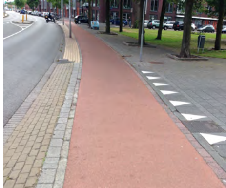
Figure 12: Tabled crossings slow cars and give priority to cyclists
