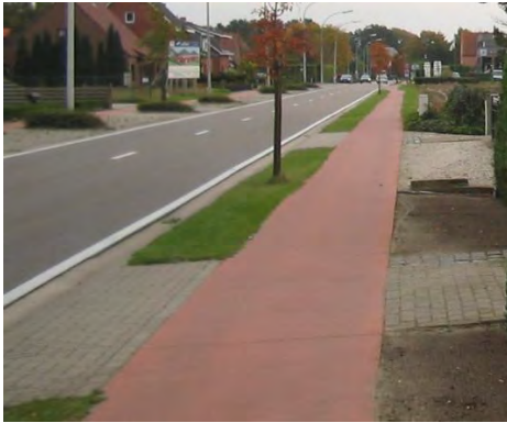
Figure 11: Cycle track continues Level across driveways
