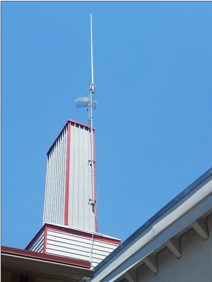
Photos of existing whip antenna and small dish, currently side mounted on the north communications tower.
