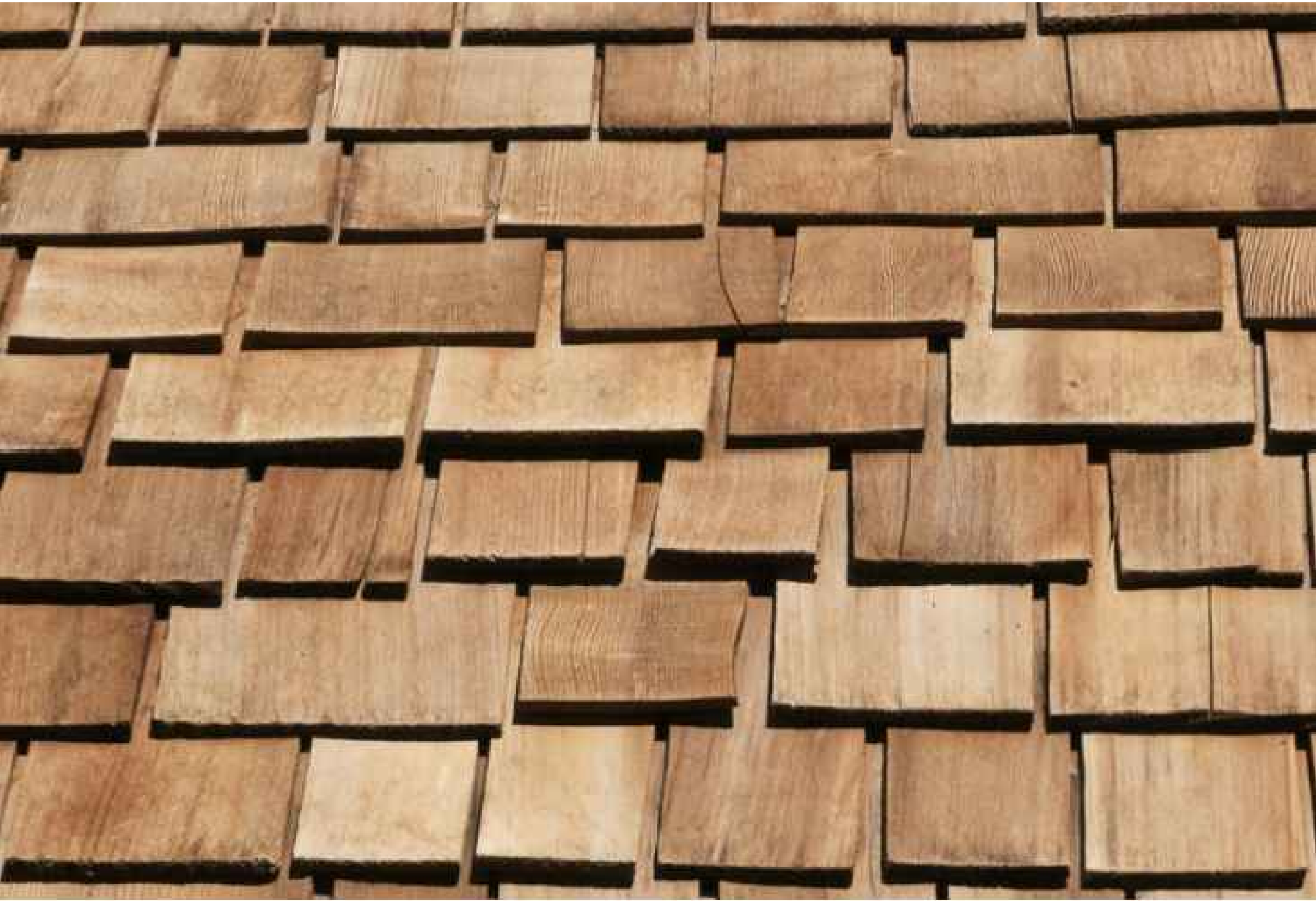
CEDAR SHAKE ROOF AT CANOPIES, OILED TO MAINTAIN BROWN TONES
