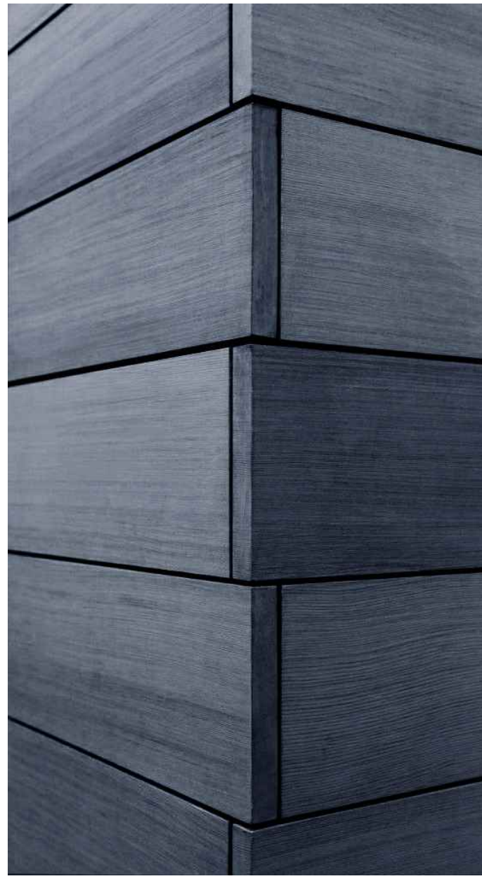
2x10 STAINED IPE RAINSCREEN MATERIAL AND CORNER DETAIL AT NEW BUILDING ENTRY CANOPY
