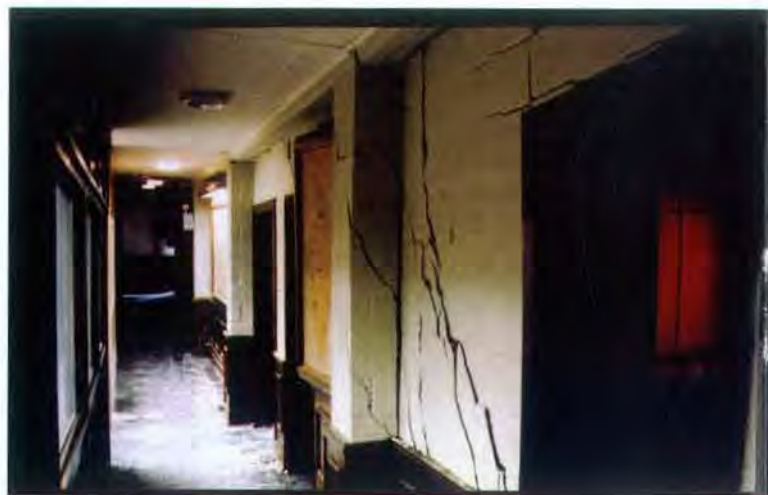
Figure 4. Building damage due to loess collapse.
